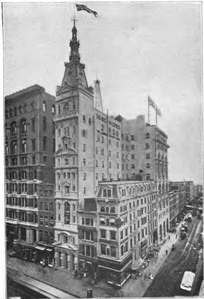
THE MAIL AND EXPRESS BUILDING. BROADWAY, SOUTHWEST CORNER OF FULTON STREET; OPPOSITE ST. PAUL'S CHURCHYARD.
